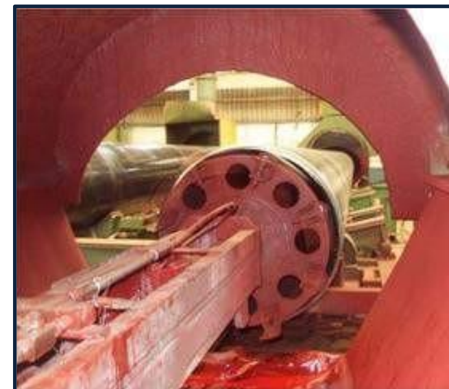
Internal Coating Application
